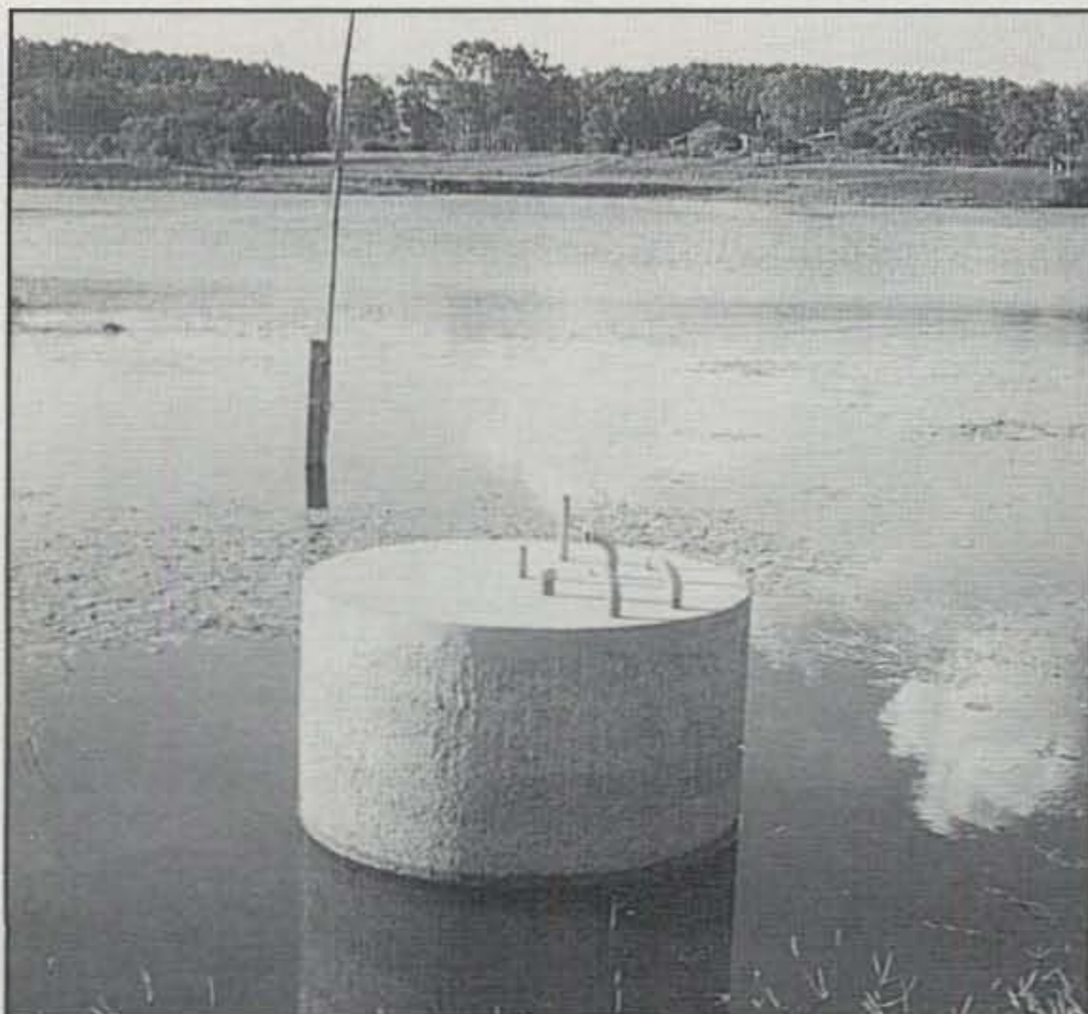
Concrete base before the tower was installed. Capped PVC pipe contains the 0.25-wavelength image wire.
